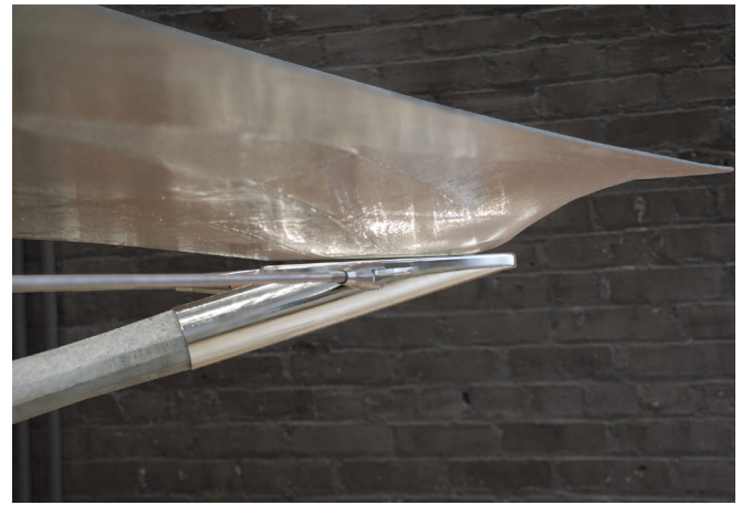
10 The glass-steel support connection beneath view © PSL.
