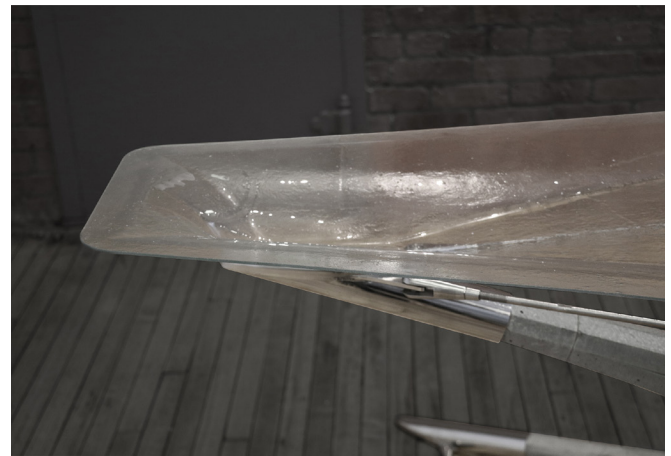
11 The glass-steel support connection above view © PSL.
