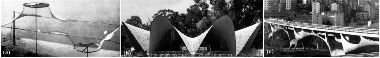
Figure 2: Minimal surface as large-scale structures; (a) Frei Otto's soap film experiment[22], (b) Los Manantiales restaurant by Felix Candela[13], (c) Bridge over the Basento by Sergio Musmeci[5].
